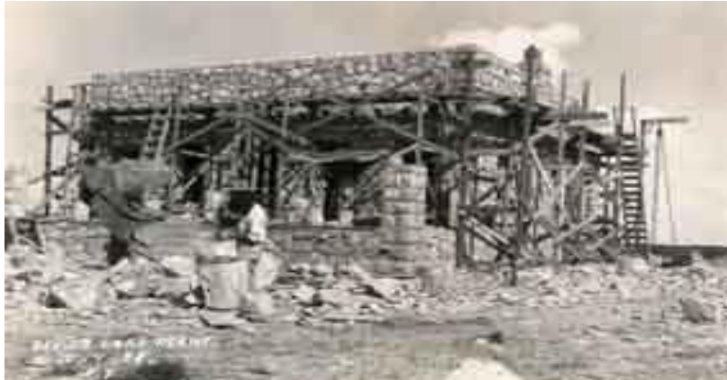
Construction of the Devils Lake Power Plant in 1928. (Photo Courtesy of Whitehead Museum)
