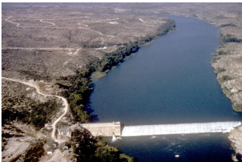
Lake Walk Hydro Plant, located several miles downstream from Rough Canyon Campground, was submerged by Amistad Reservoir in 1972.
