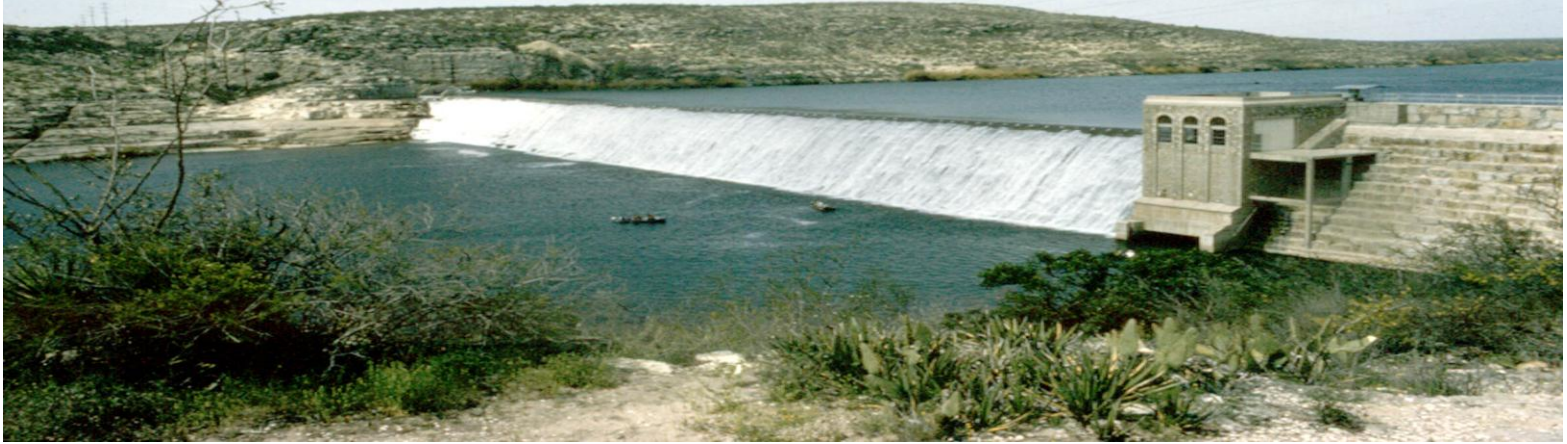
Devils Lake Hydro Plant
