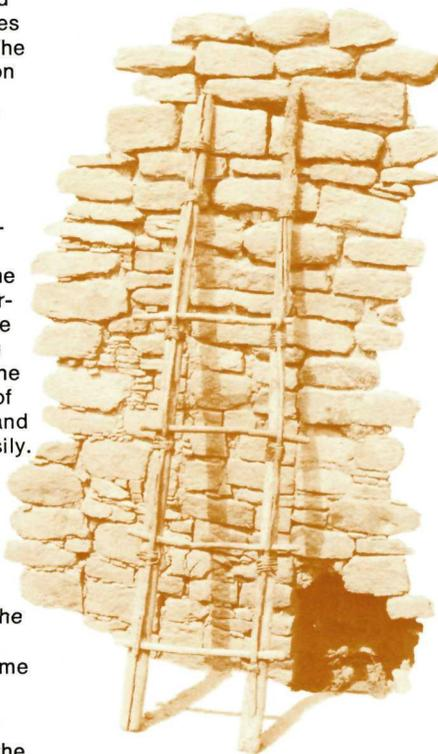
*It took a tremendous amount of labor to build these walls. All of the stones had to be carried here from several kilometers away, then shaped by hand with just another stone for a tool. As the floors and walls were added above ground, the builders probably hauled the stones up on ladders like this one. Ladders were also used by the Pueblo Indians simply to get from floor to floor. This is one of six found in the ruins.*
