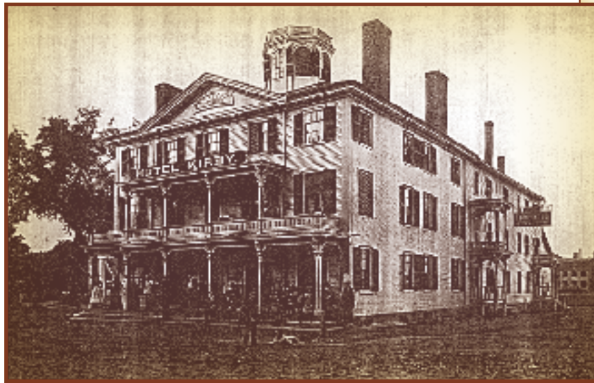
The oldest structure on the Common, the inn acquired a rear ell (as large as the original building) and a two-story porch c.1865-1875. When A.J. Kirby ran it in the 1890's, it was said to be "strictly first class."
