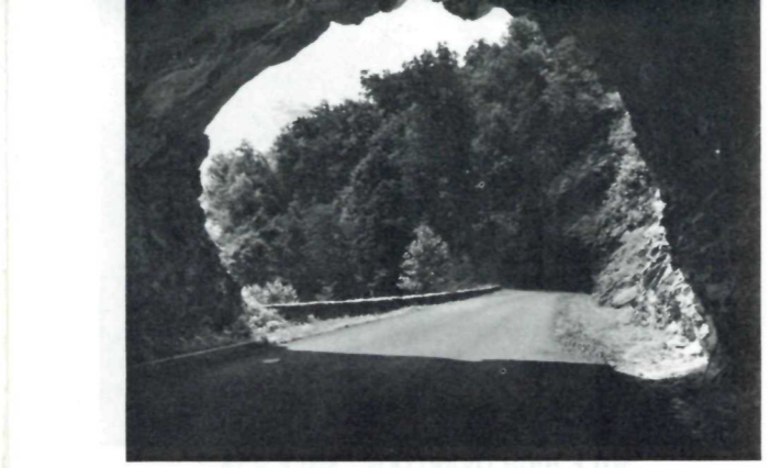
TWIN TUNNELS, MILE 344.5
