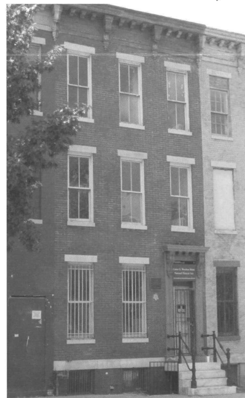
Carter G. Woodson's Home at 1538 9th Street NW, photographed in 2006 before restoration. NPS Photo.
