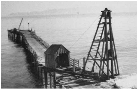
The pier with pile driver in operation.
