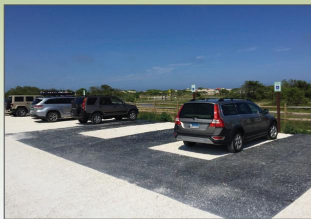
In response to accelerated shoreline erosion and greater storm impacts, Assateague Island National Seashore adopted climate-conscious solutions for beach facilities, including parking areas constructed from native clay and clamshell that can be reused in post-storm repairs.
