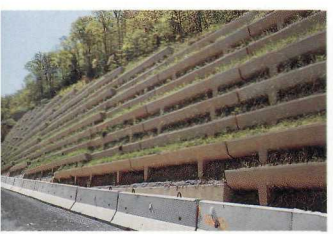
Precast Element Wall
