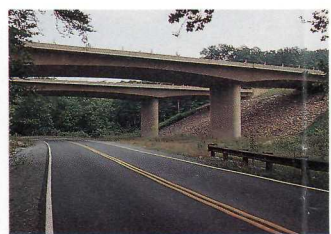
Approach Bridges/Tenn. Portal
