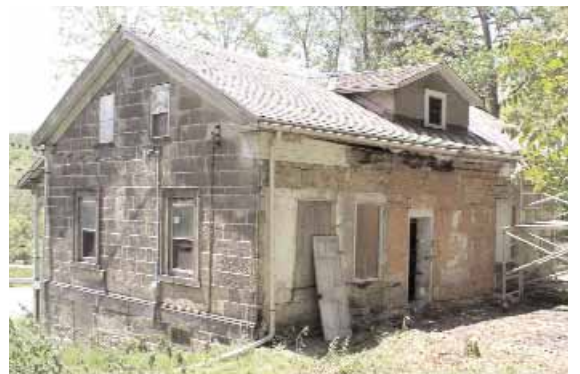
The carport addition was removed in early June, 2005. NPS Photo.
