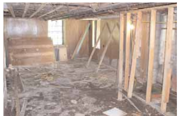
Demolition work has started in the basement. June 2005. NPS Photo.
