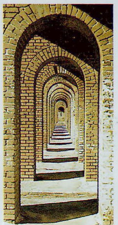
Fort Jefferson Archways
