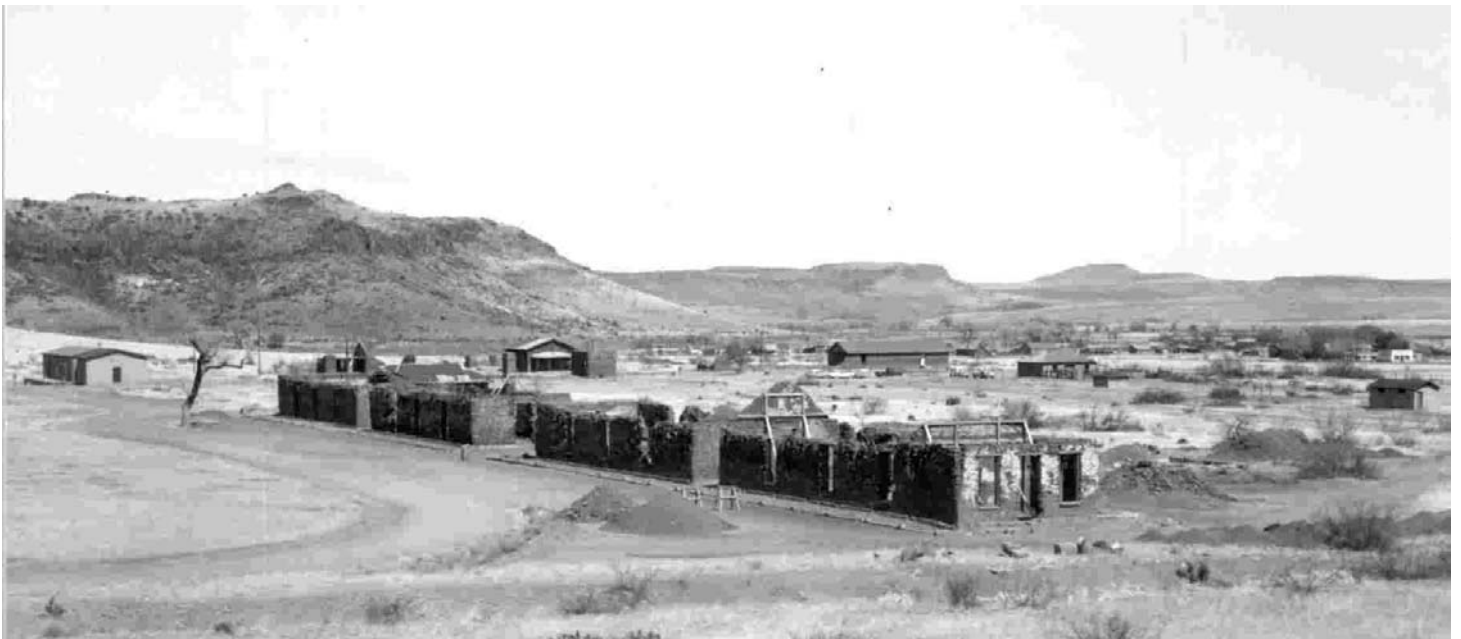
Restoration work on the Enlisted Men's Barracks began in 1963
