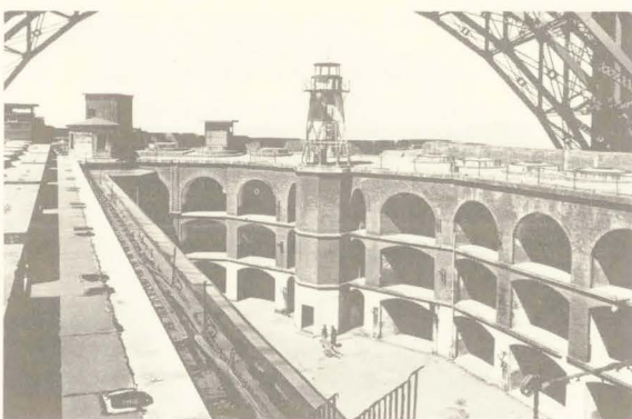
The handsome arched casemates with their intricate brickwork once housed the fort guns. There are thirty "gun rooms" on each floor.
