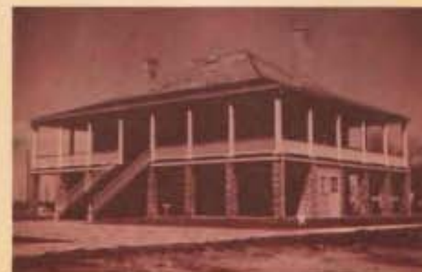
Post Hospital. Once a haven for sick or wounded Army troopers, this fine example of 19th Century architecture serves today as a Visitor Center—information service, museum exhibits and rest-rooms—for the modern traveler.
