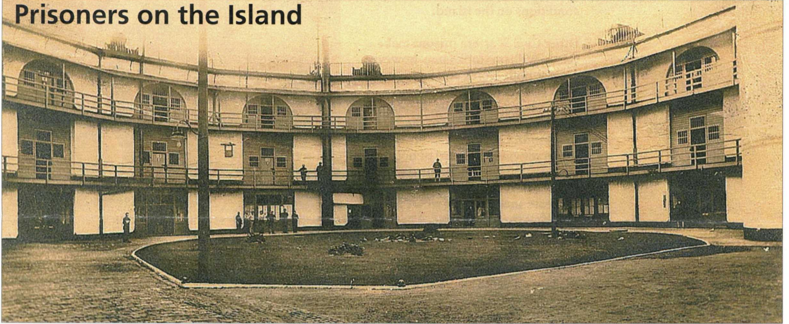
A pre-World War I postcard depicting Castle Williams' courtyard prior to the addition of the concrete-enclosed catwalks that currently dominate the Castle's interior walls
