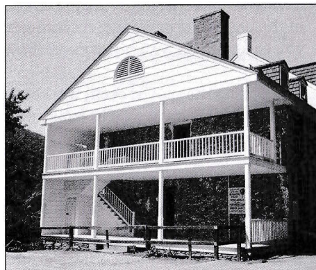
Harper House before and after renovation. (NHF10, NHF1984, Modern Photo Collection, Harpers Ferry NHP)
