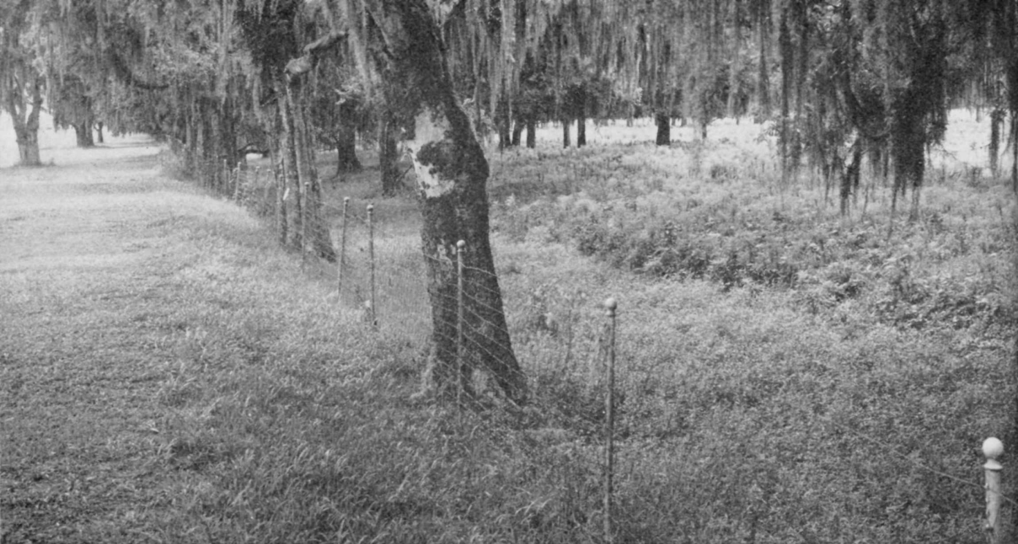
The remains of the old dry millrace, known as the Rodriguez Canal, behind which the Americans erected their mud earthwork, may still be seen at Chalmette National Historical Park. The course of the ditch is just beyond the fence which it parallels.
