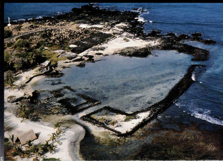
'Ai'ōpio fishtrap was constructed of lava rock by Hawaiians. Fish swam into the bay at high tide and were trapped inside the walls as the tide fell.
