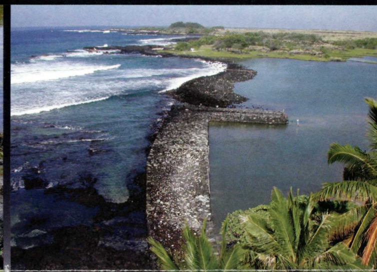
The kuapā, or rock wall, now being reconstructed, separates Kaloko fishpond from the ocean.
