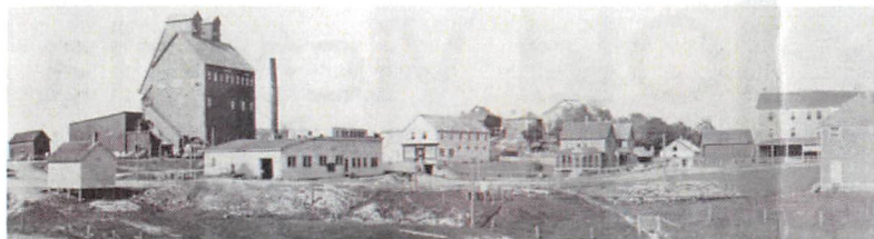
The Victoria Mine, after 1916, from left to right: shaft house, steam plant, company store, captains house, big boarding house, and company office.
