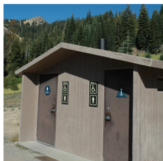
Sulphur Works accessible restroom
