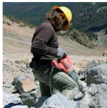
A trail crew member splits stone for relocation to a lower section of trail
