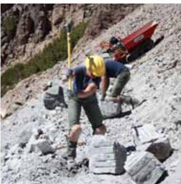
A trail crew member shapes stone to construct a retaining wall
