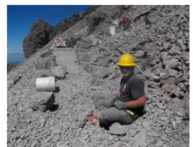
A trail crew member prepares to place a stone on a steep switchback.
