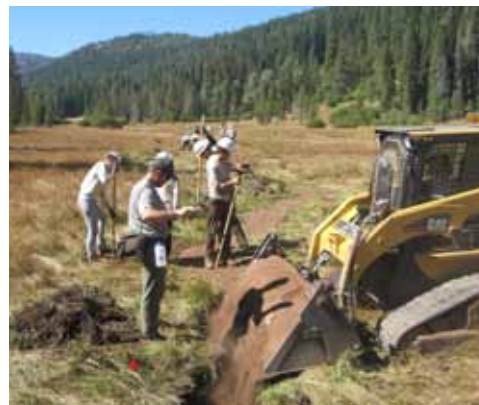
Staff fill, shape, compact, and replant downstream
