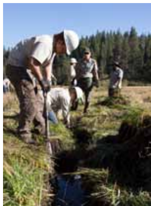
Cutting overhanging walls
