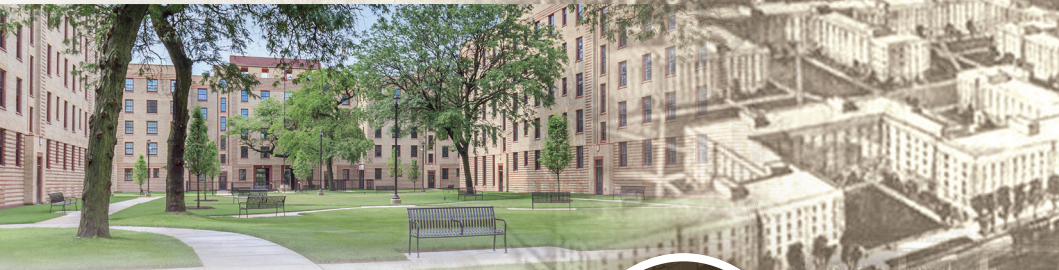
Michigan Boulevard Garden Apartments, now "Rosenwald Courts" in Chicago. Current image on left, ca. 1929 image on right.
