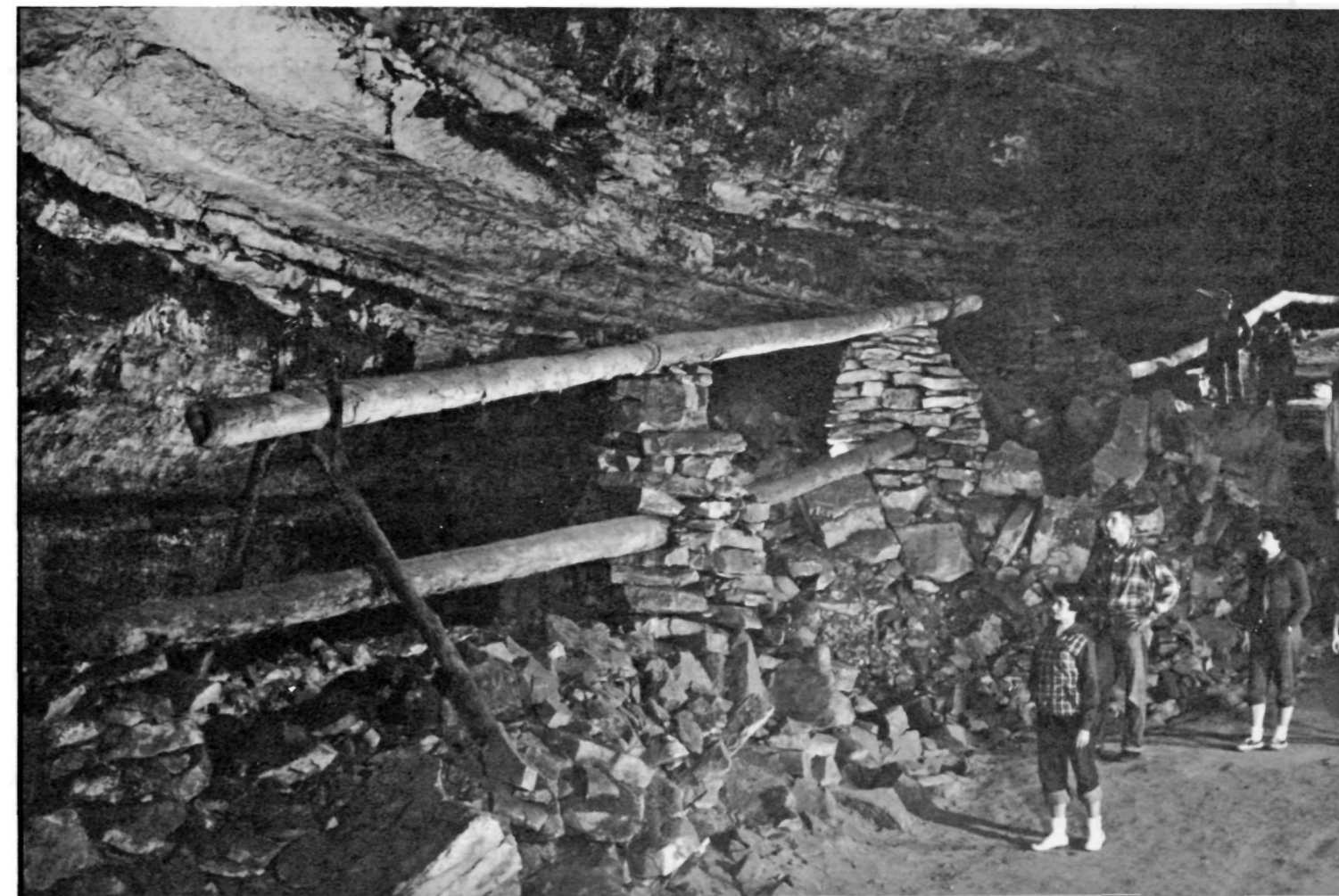
Wooden pipes used in saltpeter operations in War of 1812.
