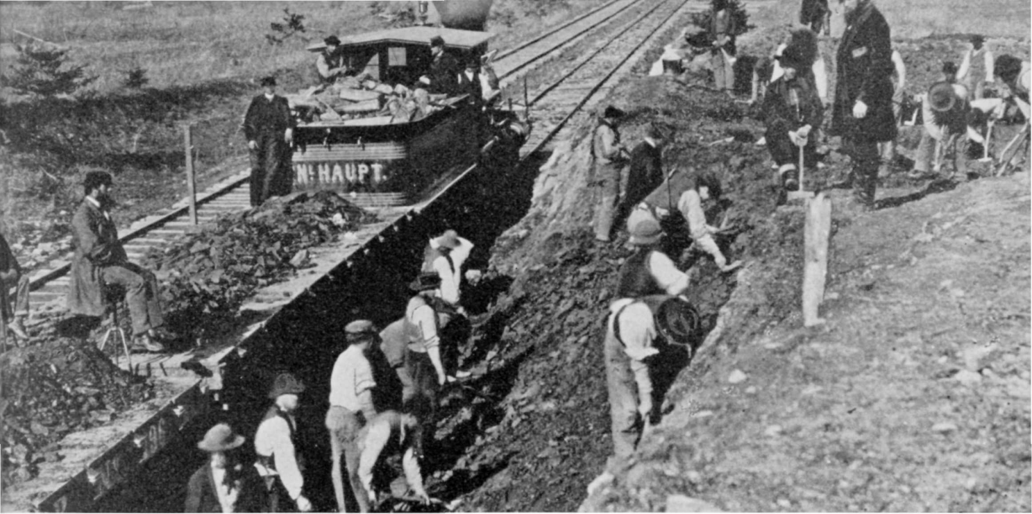
Wartime Brady photograph of the railroad near Bull Run. General Haupt is seen inspecting the work of his Federal Construction Corps. (Signal Corps U. S. Army.)
