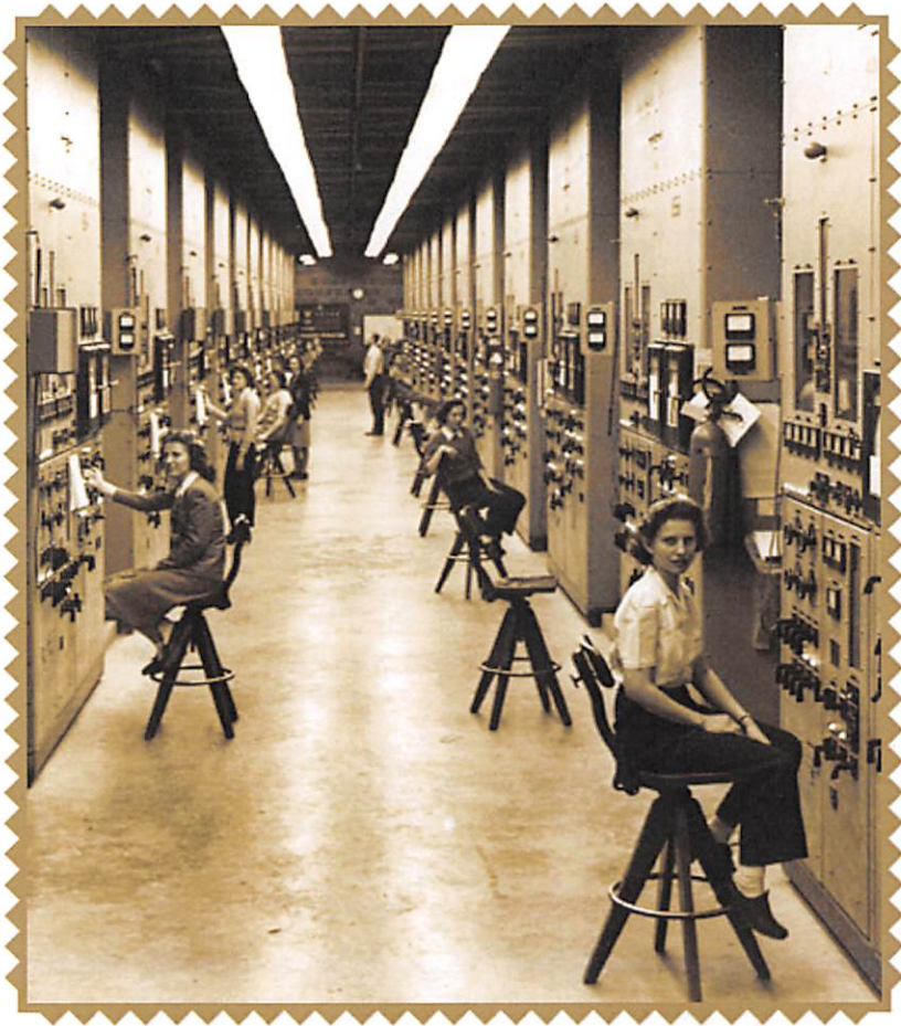
Control panels and operators for calutrons at the Y-12 plant.
