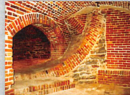
Basement Dome Support
