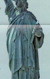
Weight of steel: 250,000 lbs. Thickness of copper: 3/32" (two pennies)
