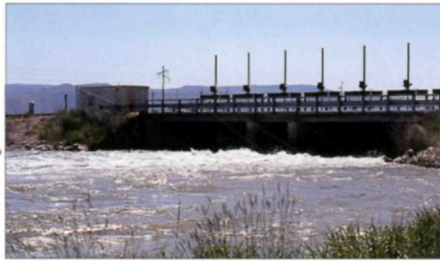
The Outlet Canal control structure regulates water levels in the marsh.
