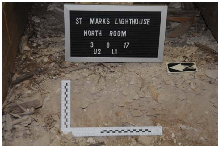
Figure 3-surface below floor, NW corner
