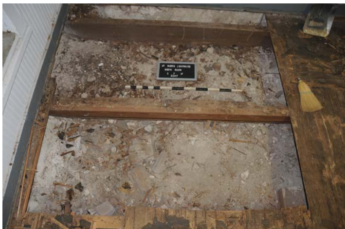
Figure 1 removing the floor in room's NW corner
