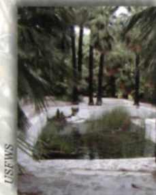
Abandoned concrete pools at Moapa Valley.
