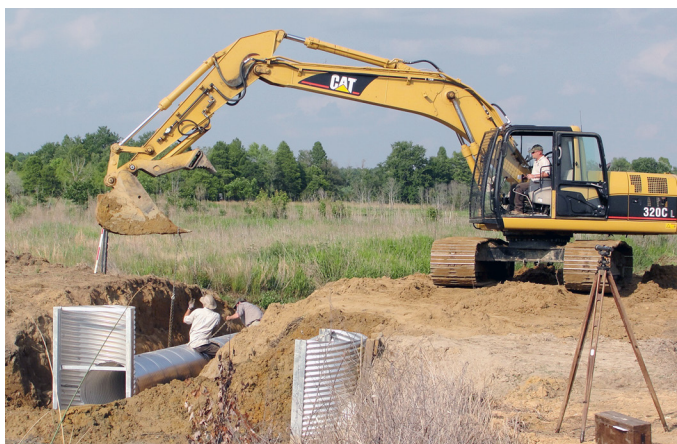
Installing a water control structure by Marc Epstein/USFWS
