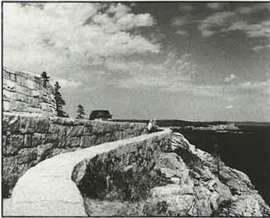
The Olmsted Center prepared rehabilitation guidelines for the Historic Motor Roads at Acadia National Park.
