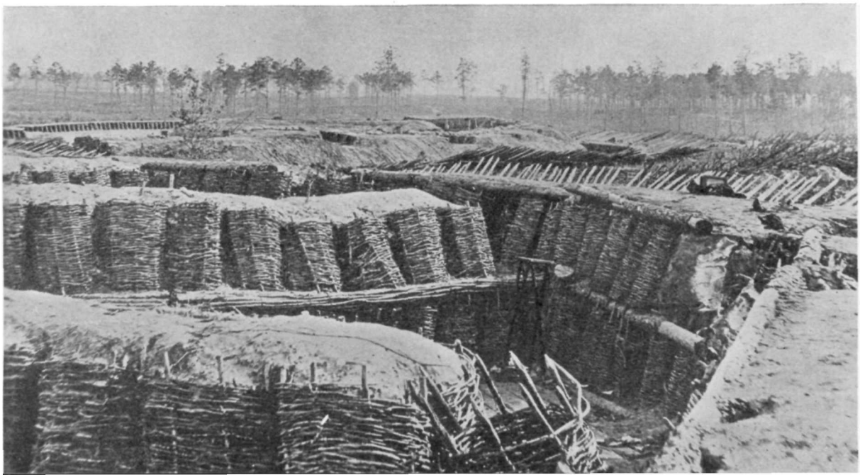
Trenches used by the Confederates in the defense of Petersburg. Note the use of rolls of wickerwork, or gabions, to line the sides of the trenches. Courtesy Signal Corps, U. S. Army.
