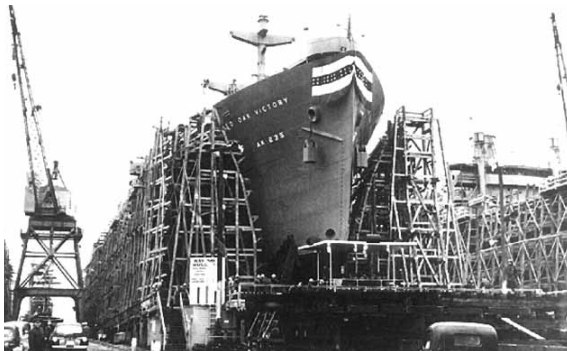
The SS Red Oak Victory being constructed, Richmond Museum of History Collection.
