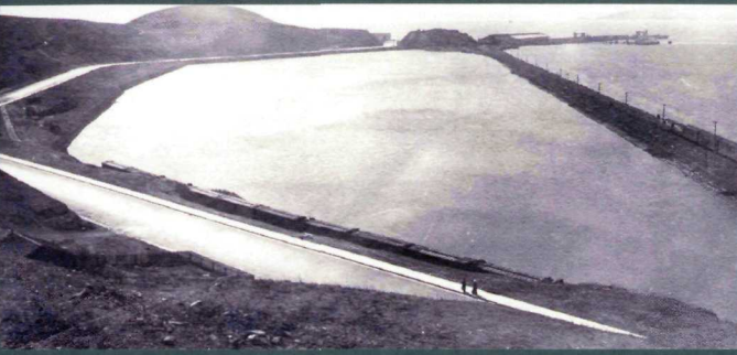
Lagoon formed by Santa Fe rail line (now the home of Miller/Knox park)
