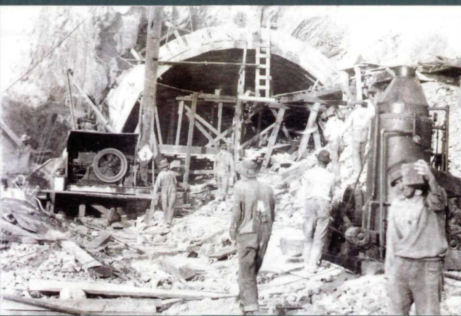
Building the Ferry Point Tunnel in 1914
