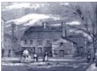
7 310 ½ Essex Street, the Jonathan Corwin House. Pencil sketch, 1841, by Edward C. Cabot.
