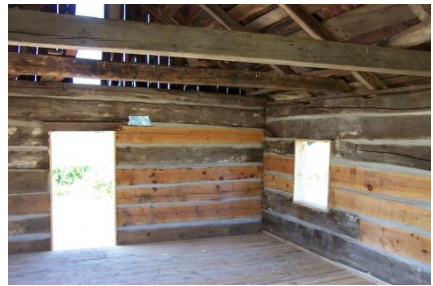
Inside the Shalda Cabin during restoration
