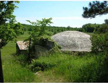
Treat Garage from walkway to the house 2007
