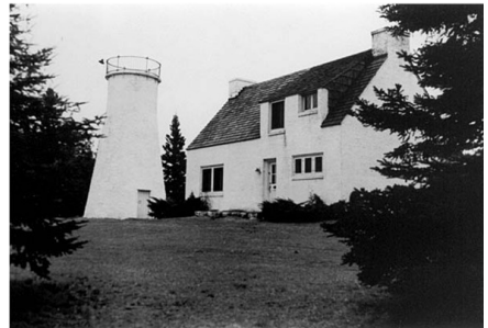
Old Presque Isle Lighthouse built to the same specifications as the 1839 SMI Lighthouse.
