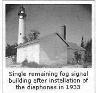
Photo courtesy of HABS/HAER Single remaining fog signal building after installation of the diaphones in 1933
