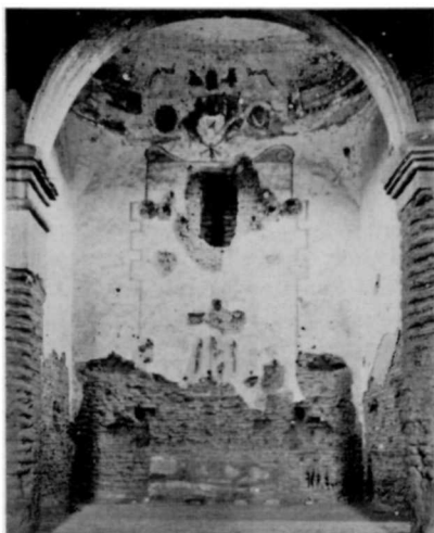
North wall of sanctuary as it is now.
