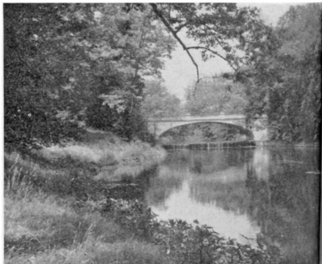
Crum Elbow Creek where it is crossed by the entrance drive.
