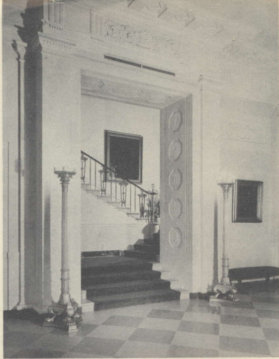
Entrance Lobby and Main Stairway
