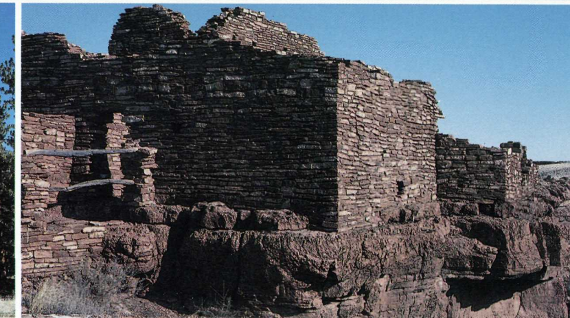
Standing on the edge of a 3/4-mile-long earth crack is the ruin known as Lomaki, or "pretty house." Earth cracks, resembling canyons, are fractures in the Kaibab limestone usually associated with earthquakes or volcanoes.
