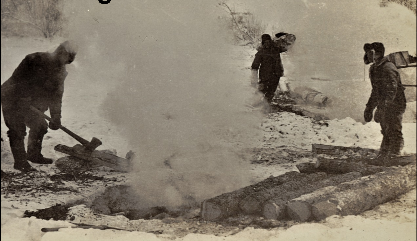
Miners cutting wood to feed the fire in their prospecting shaft, 1898. After ‘burning down’ through frozen ground, they will continue using fire to ‘drift’ horizontally to reach the richest gold deposits. Glass photographic negative, author’s collection.
