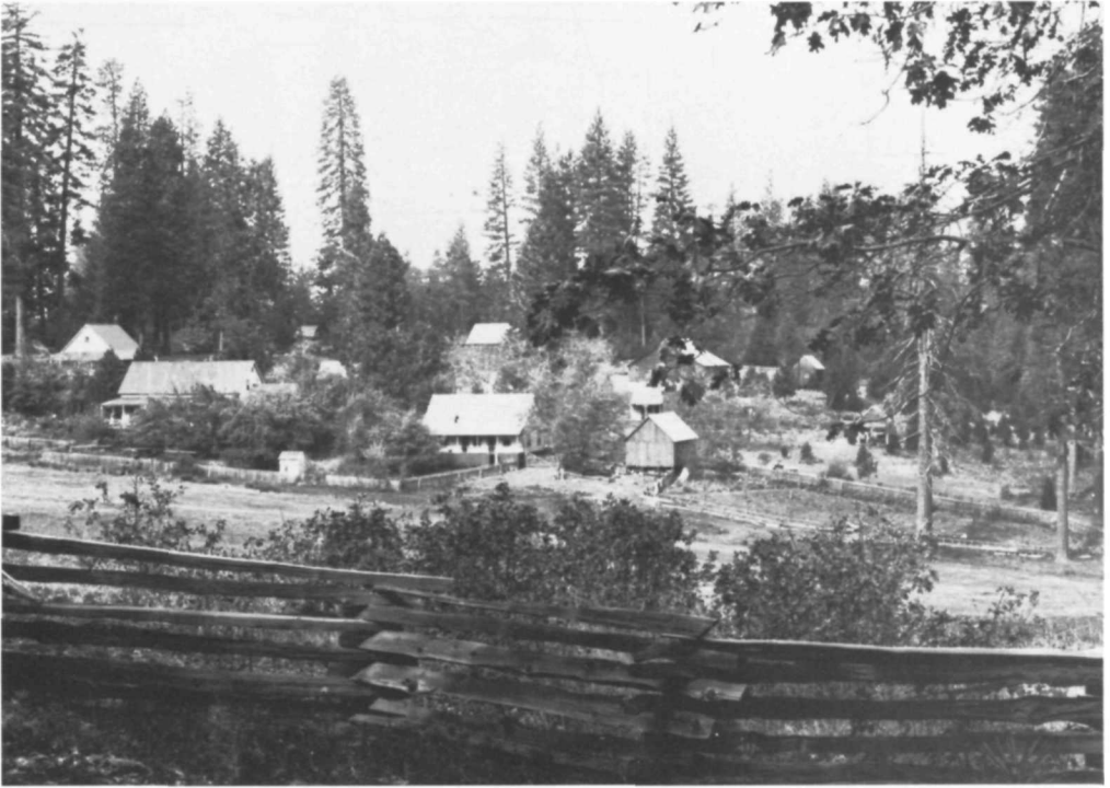
The western portal, Crocker's Station, 1901
