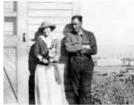
National Park Service photograph
