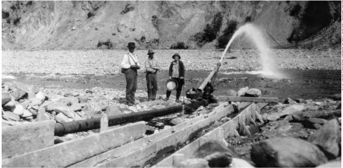
Joe Quigley, Johnny Busia, and Fannie Quigley observe hydraulic placer mining on Moose Creek, 1922
