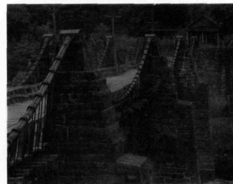
Oldest suspension bridge in U.S. designed by John A. Roebling, engineer for the Brooklyn Bridge, New York.
