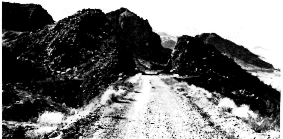
Earthen or rock fills (foreground) and cuts (center) are common features of abandoned railroad grades.
