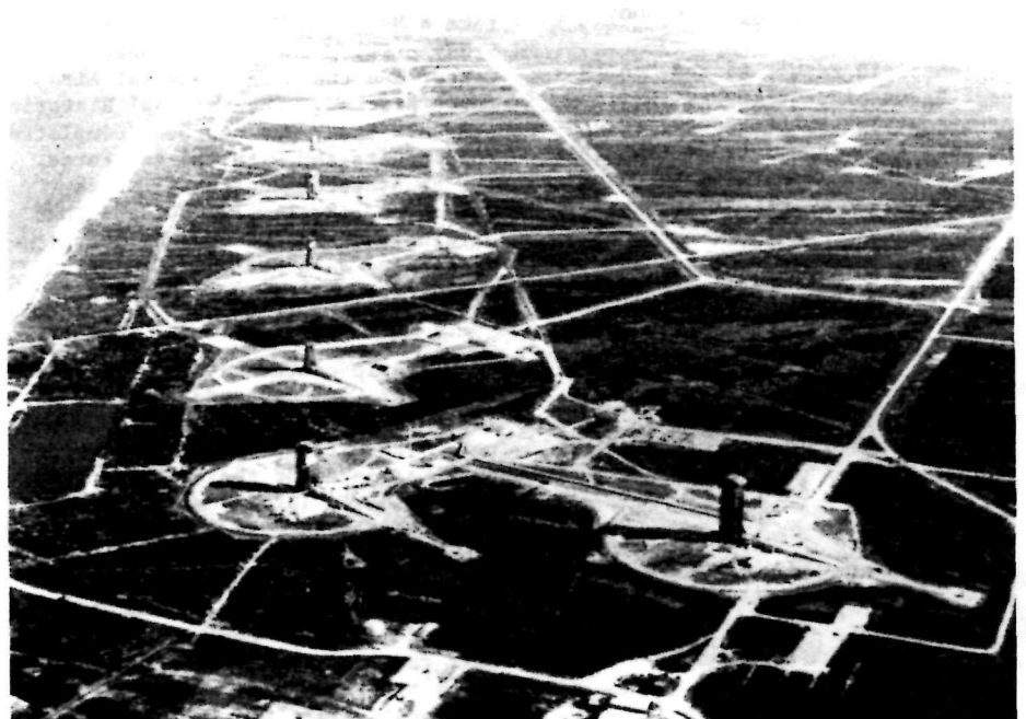
Aerial view of "Missile Row," looking north in 1964.
